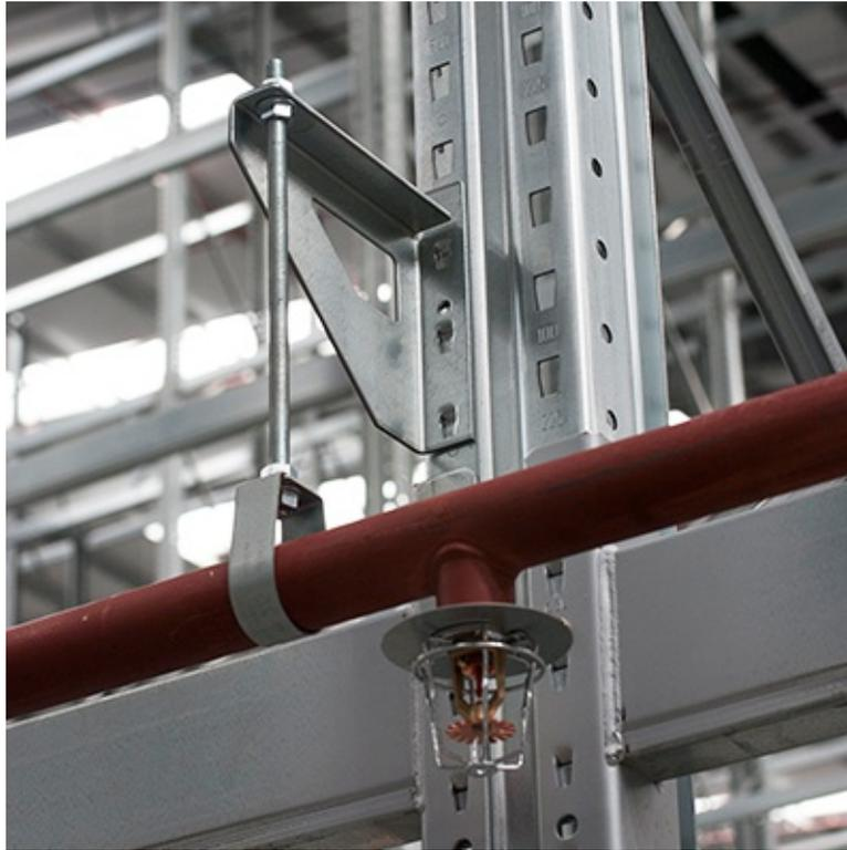
However, all this relies on the pipework that carries the water or air/gas being correctly installed and remaining straight and true. If the pipework becomes bent and out of shape to such an extent that the water- in the case of wet-pipe sprinkler system, or gases or compressed air - in the case of dry-pipe systems –the consequences can be devastating. Even if no lives are lost, or injuries sustained, the loss of stock through fire or water damage can and does destroy businesses.
